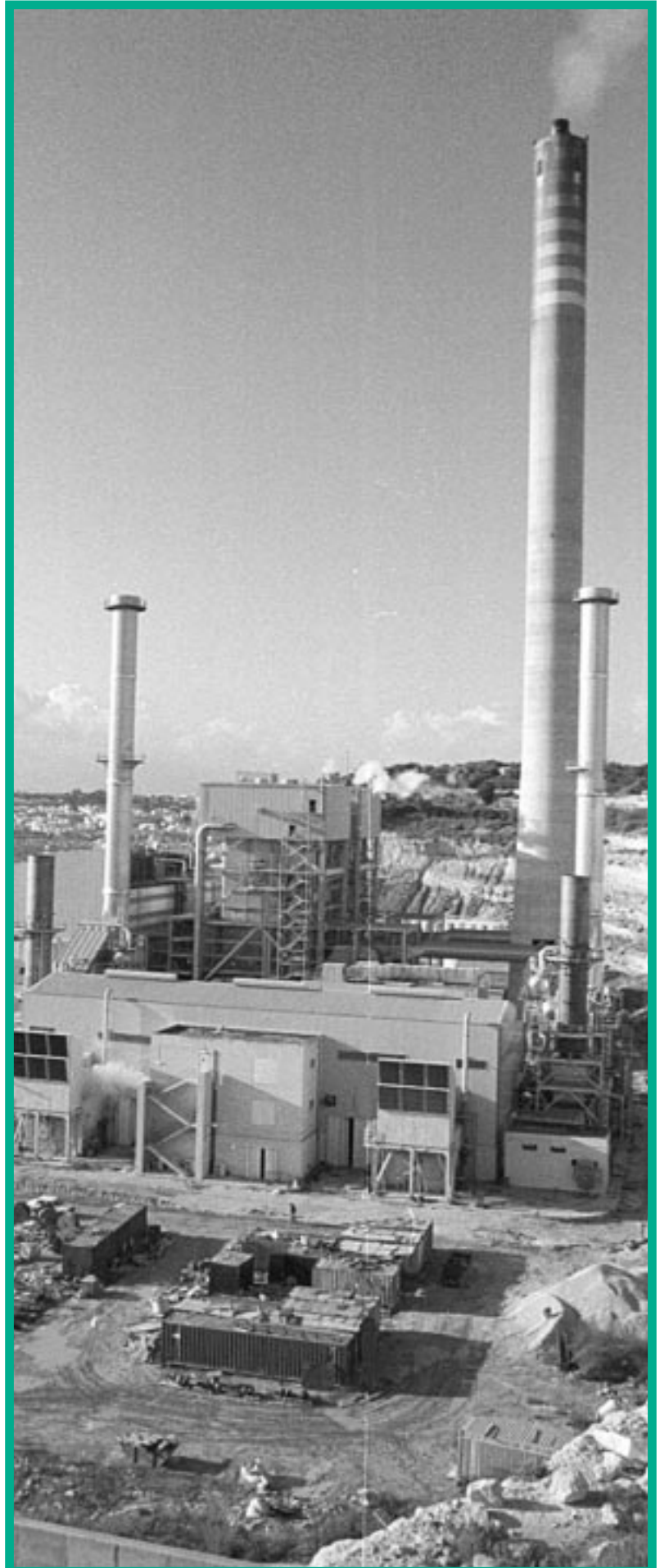
Delimara power station to adapt to EU standards on dust emissions by 2005
